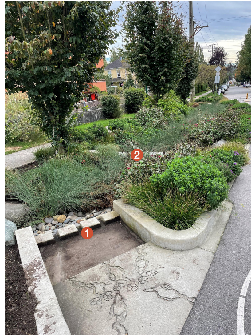
Figure 38: Bioswale on Woodland Drive in Vancouver, BC
