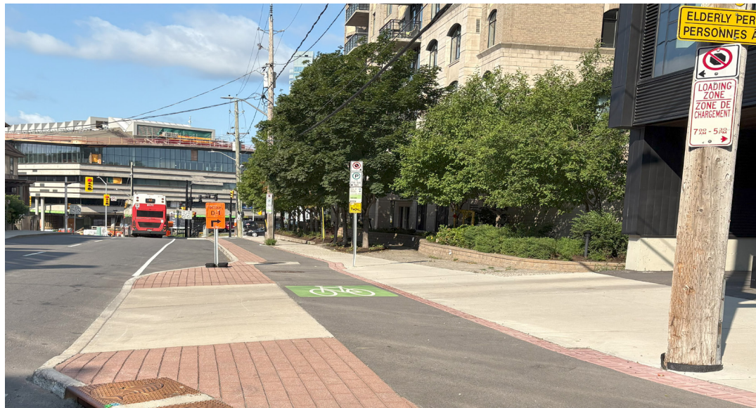
Figure 47: Continuous sidewalk and cycle track across driveway, with ramp limited to width of amenity zone and minimized turn radii
