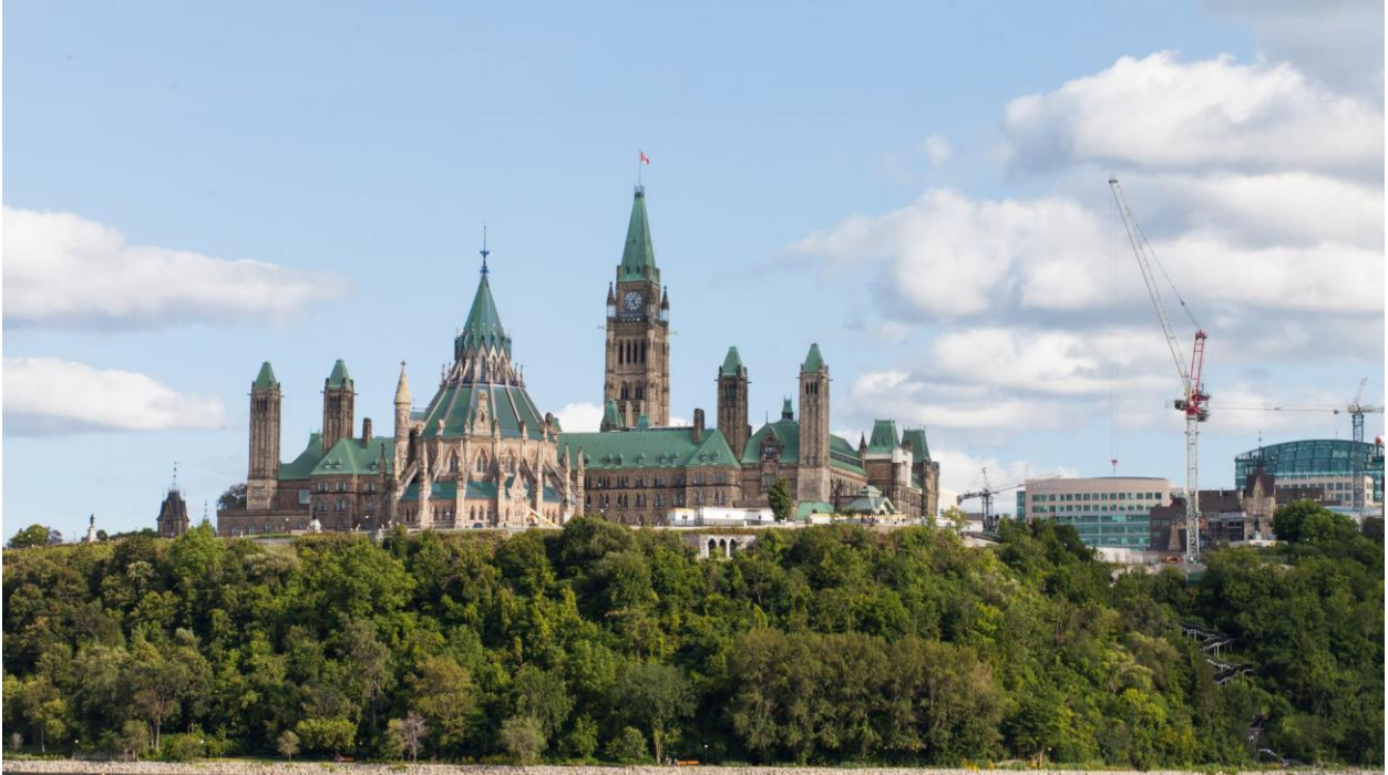
Existing view of Centre Block from the Canadian Museum of History looking toward Library of Parliament.
